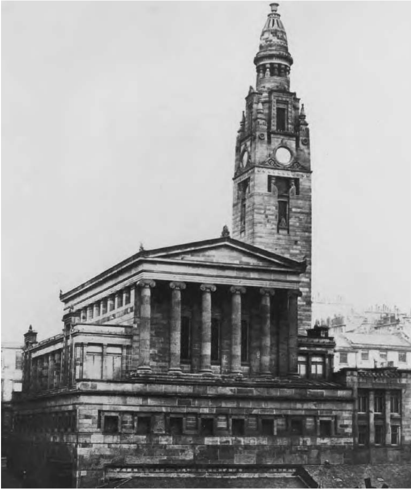
Plate 201 Alexander Thomson's St Vincent Street church, Glasgow (1859) , showing the Egyptian pylon-forms in the tower and breaking through the side-walls of the aisle above which is the clerestorey of square columns. Note the two Cherubim facing each other in the T-shaped opening in the tower beneath the clock. Photograph of c.1890 (RCAHMS GW.2017).
